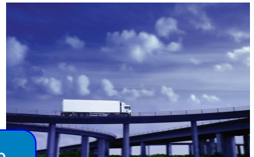
Fig. 7.2 The internal forces in the beams of the overpass shown vary as the truck crosses the overpass.
