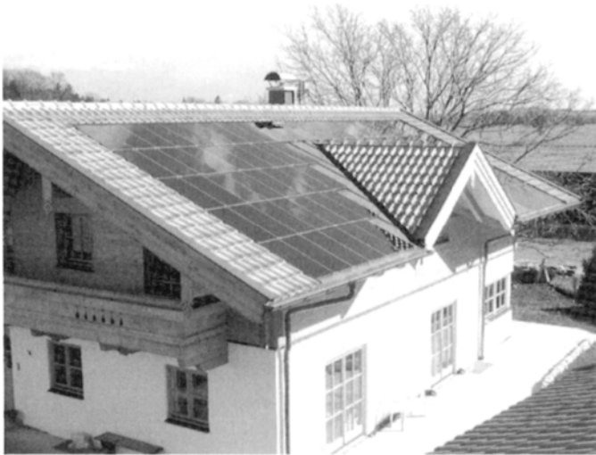
Figure 27 Installation of CdTe modules on a private residence roof.
