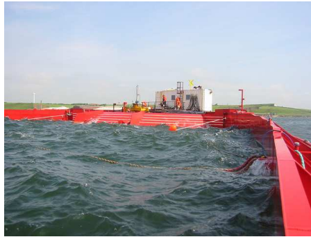
Fig. 18.4. Wave Dragon seen from reflector, prototype 1:4½.
