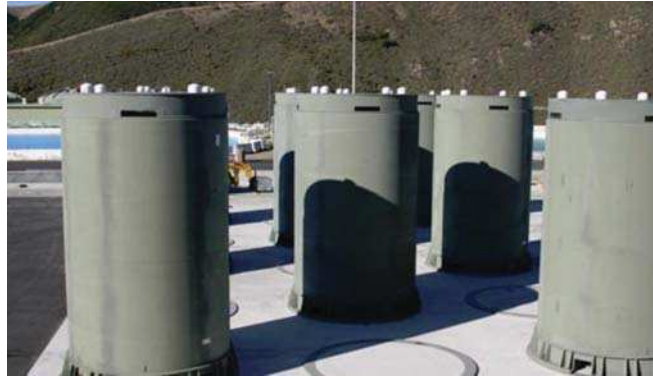
Figure 5.13 Typical dry cask storage containers. (Courtesy of the U.S. Nuclear Regulatory Commission.)
