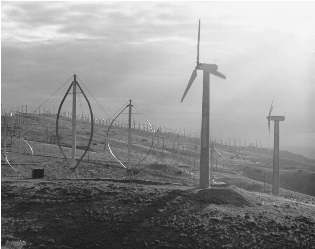
FIGURE 8.11.2 Wind farm both horizontal-axis and vertical-axis turbines.
