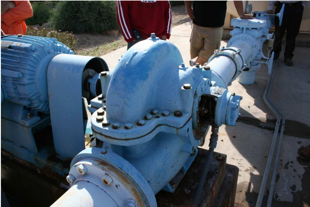
Split-Case centrifugal pump.
