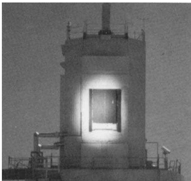
FIGURE 17.4 Experimental 1050°F thermal receiver tower for Solar-II power plant. (From: DOE/Sandia National Laboratory.)
