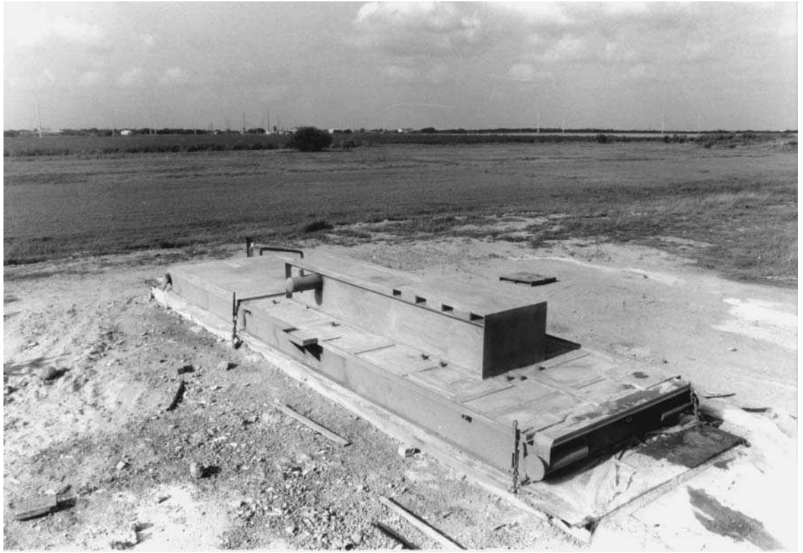
FIGURE 23.2 Typical skid design with concrete fill.
