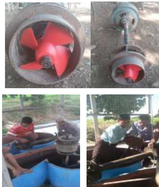
Figure 7. Installation Process of Turbine
