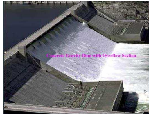
Figure 1. 11 Concrete gravity dam with overflow section
